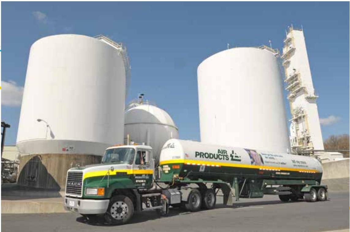
Oxygen is either produced at large cryogenic air separation plants and then transported by tank truck to a customer's site or, in some cases, it can be generated directly on location.
