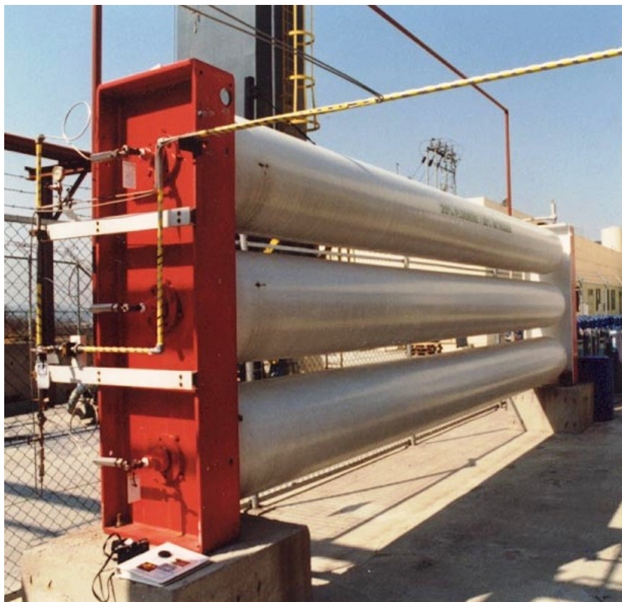
Figure 2: Typical Ground Tube Installation
